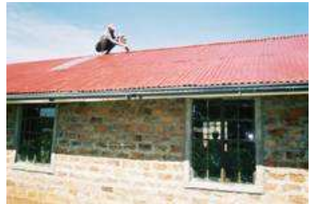
Painting the roof of the school
