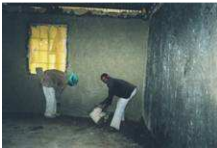
Plastering the classrooms
