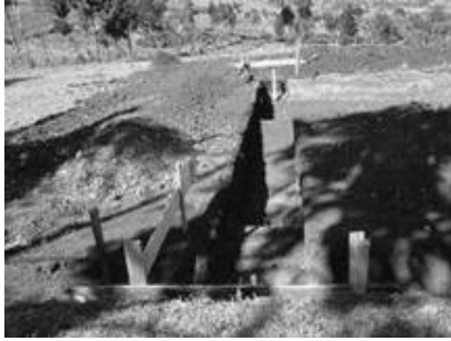
Foundations for the new medical centre
